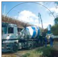
Ready-mixed concrete plants
